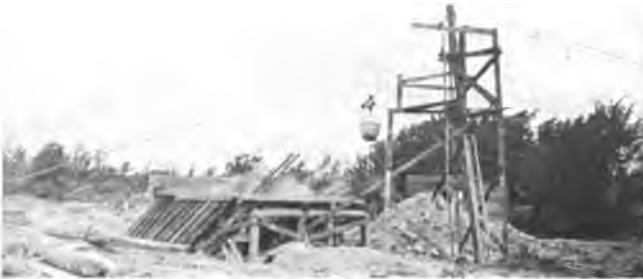
B. STARTING SHAFT SINKING AT ST. LOUIS MINE.
